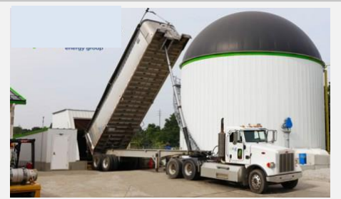
Figure 1: An anaerobic digester converts food waste to biogas via biological processes.
